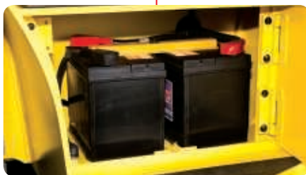
Maintenance Free Batteries
